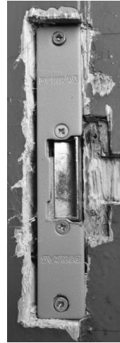
FIGURE 6-2: THE ELECTROMECHANICAL DOOR LATCH
